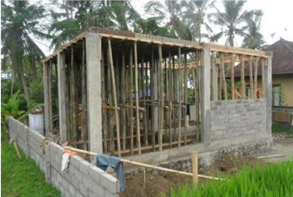
Siddharlo's Guest House under construction
